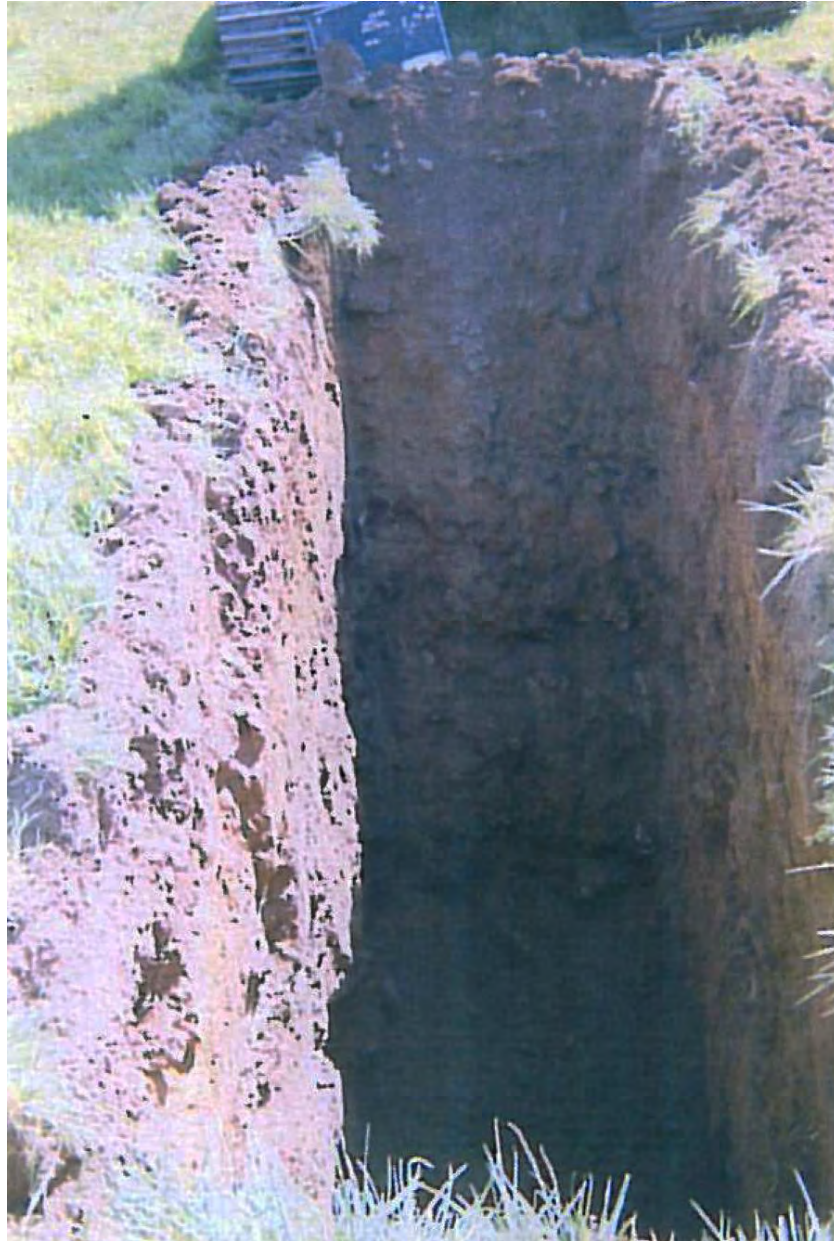
TP A10 Digging Face 2
