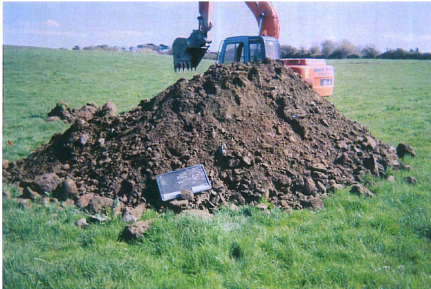
TP A10 Side Wall
