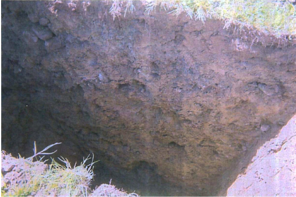
TP A13 Side wall 1
